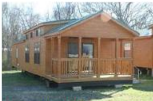
741 - Exterior with clerestory dormer
